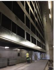
The tunnel portals are equipped with four 55-ton hurricane flood gates, designed to withstand hydrostatic flood forces for a design water elevation of 22.6-ft based on the 500-year design storm event. This feature -already activated 3 times as of mid-2022- could help avoid up to \$1bn in potential flooding costs, and the city of Miami has gone on to broaden its Climateresilience boosting approach, and joined the C40 resilient cities network...
